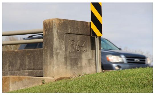
Historic Fabric Photo 2: Detail of endpost and concrete barrier and aluminum tube railing on approach spans.
