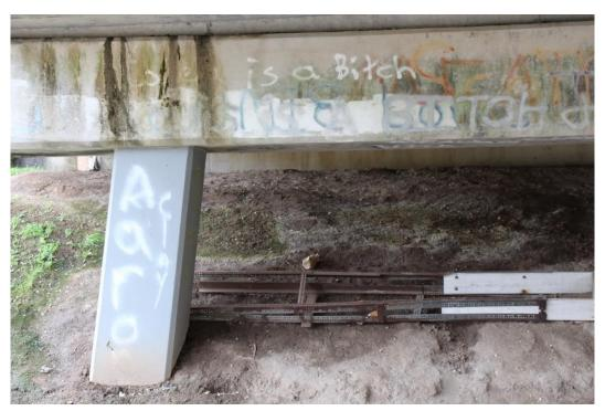
Condition Photo 14: Bent 2, concrete bent cap, and pile columns showing graffiti, water staining, and coating.
