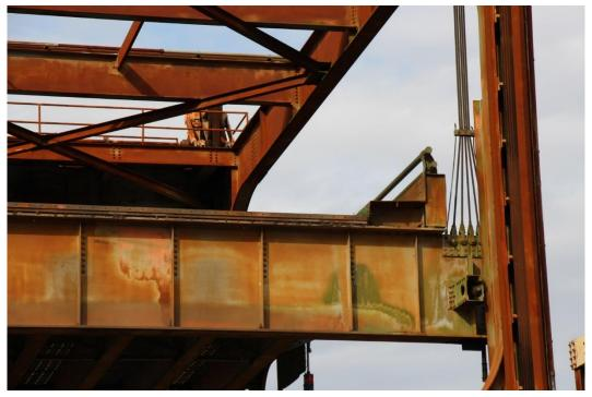
Condition Photo 4: Vertical lift span at lift girder, showing failed paint system as well as the condition of the wire ropes that attach to the lift girder and the condition of the guide tower.
