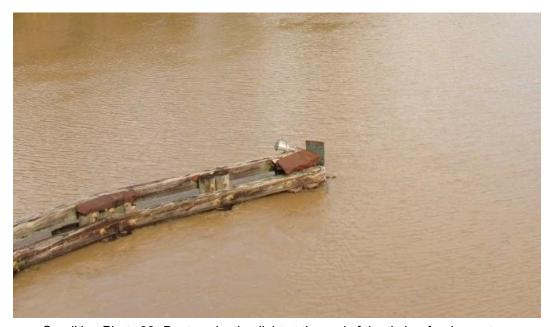
Condition Photo 22: Bent navigation light at the end of the timber fender system.
