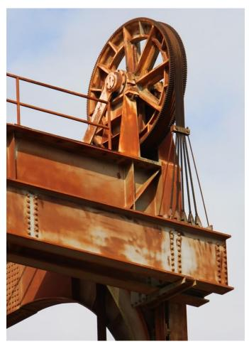
Condition Photo 5: Sheave and wire ropes on the corner of the vertical lift span.
