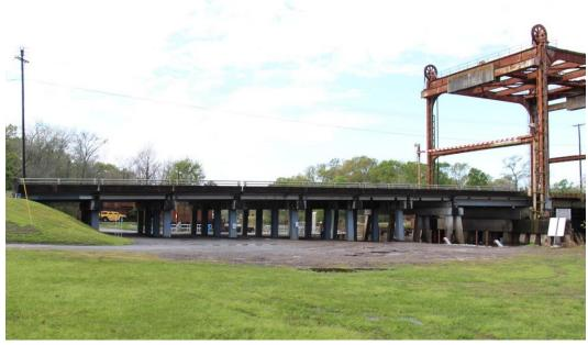
Historic Fabric Photo 1: Approach spans on the northeast side of the bridge, including the cast-in-place concrete slabs and steel I-beam spans supported on concrete piers and abutment. The photo also shows the steel traffic barrier gate and supporting towers adjacent to the lift span.
