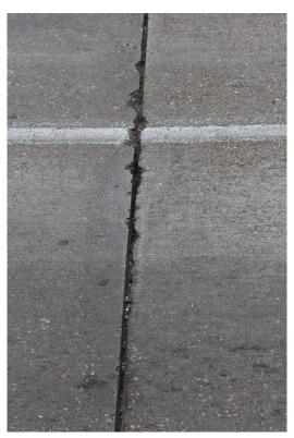
Condition Photo 18: Concrete spalling along relief joint on approach span.
