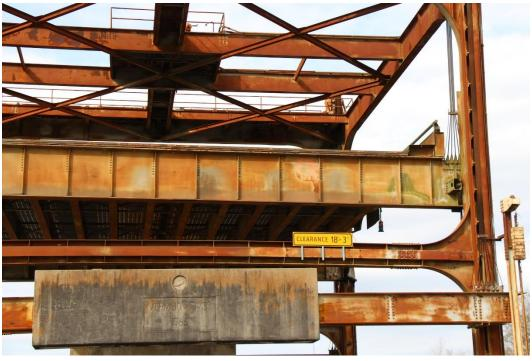
Condition Photo 8: Condition of longitudinal steel stringers framing into the end lift girder.
