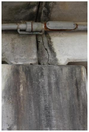
Condition Photo 15: Cracking of the concrete slab haunch at the concrete bent cap. Also note condition of expansion joint in metal conduit for electrical cable.
