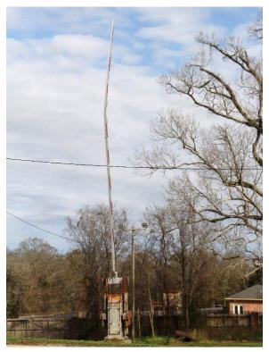
Condition Photo 23: Bent traffic warning gate arm and paint system failure.
