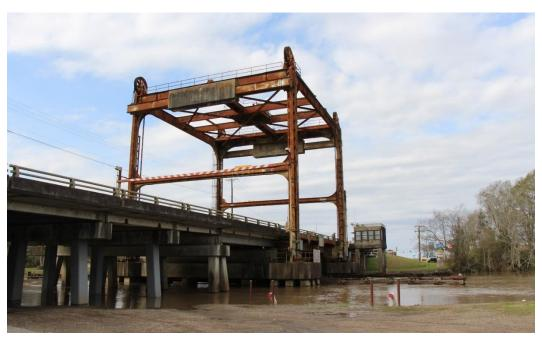
Character-defining Feature Photo 1: Design and construction of a vertical lift span with central drive machinery. The operating machinery, located at the center of a platform, drives the four sheaves on each corner of the lift towers. Note the location of the operator's house on the northwest quadrant of bridge, which is part of the historic fabric, not a character-defining feature.
