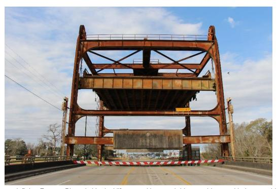
Character-defining Feature Photo 2: Vertical lift span with central drive machinery, with the movable span open, with steel barrier gates and concrete counterweights lowered.
