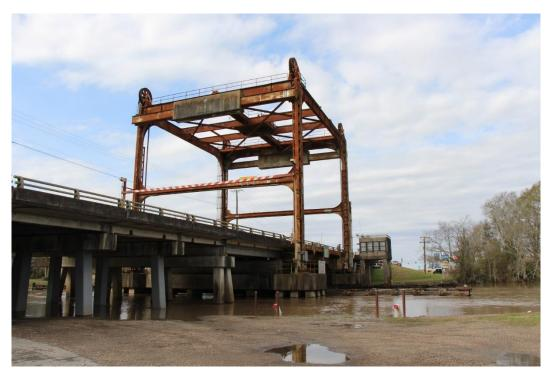
Condition Photo 13: Overview of vertical lift span showing water staining on the substructure units and the concrete piles, several of which are surface-coated.
