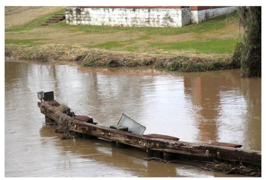
Condition Photo 21: Decay and heavy vegetation growth and debris in timber fender system.
