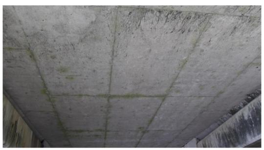
Condition Photo 16: Cracking and efflorescence of the underside of the cast-in-place concrete approach spans.
