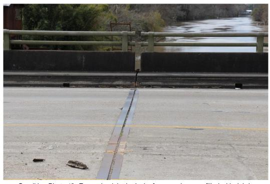
Condition Photo 12: Expansion joint in deck of approach spans filled with debris.
