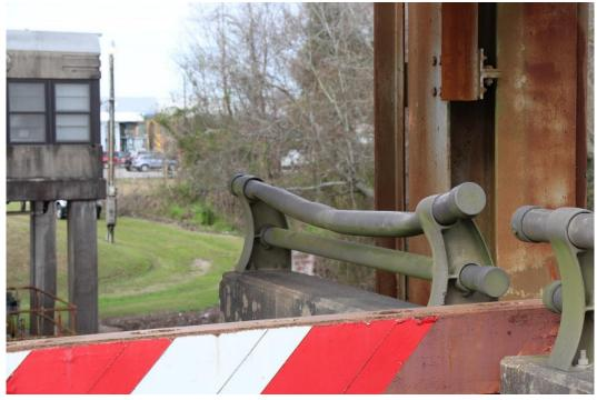
Condition Photo 20: Damaged aluminum tube railing at lift tower in northwest corner of lift span.
