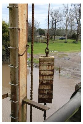
Condition Photo 9: Corrosion and paint failure on the counterweight and tower for the traffic barrier railing, typical for four towers and counterweights.
