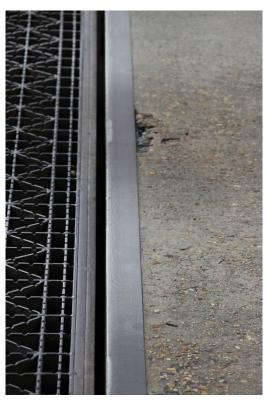
Condition Photo 19: Spalled concrete at an open joint between the lift span and the approach span.
