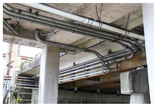
Condition Photo 17: Paint system failure on the steel approach spans.
